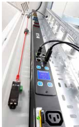
Eaton EMP Gen 2 daisy chained on rack PDU
